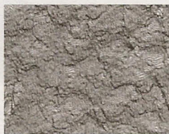
CSP 7 (heavy abrasive blast)
