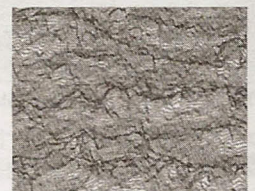
CSP 9 (heavy scarification)
