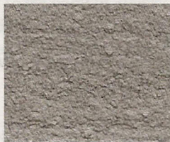
CSP 4 (light scarification)
