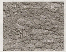
CSP 6 (medium scarification)
